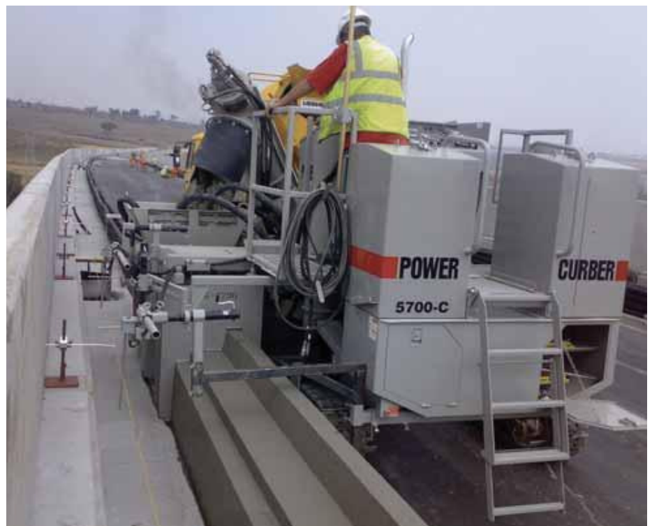
High speed rail application, pouring encasement over electrical conduit.
