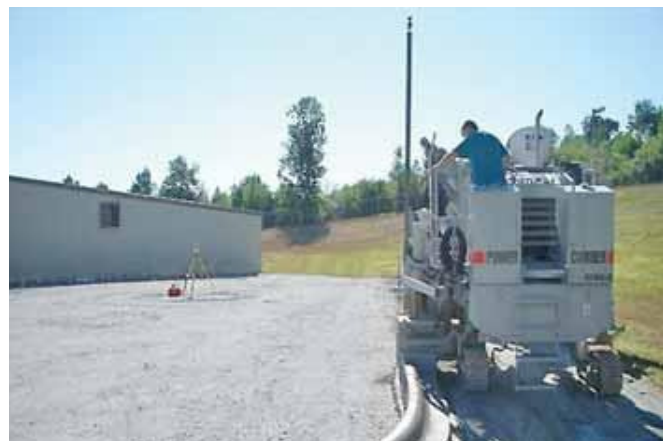
Pouring curb & gutter with 3-D (stringless) control.
