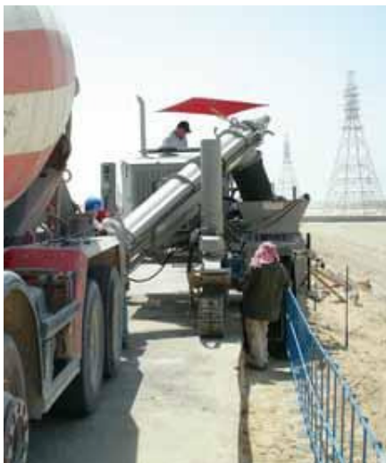
Barrier below grade with rebar.
