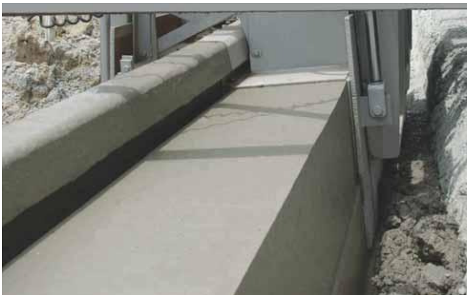
Slotted drain poured below grade.
