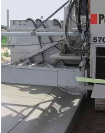
Monolithic curb, gutter, and sidewalk.
