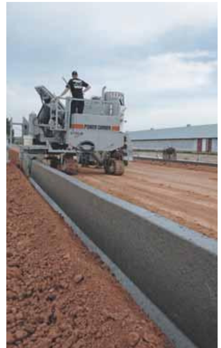
Poultry house foundation poured over trench.
