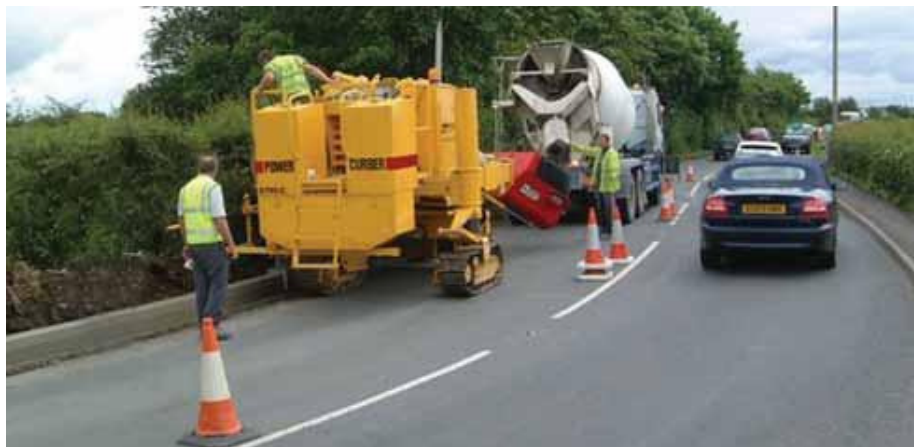
Single lane pouring minimizes traffic interruption.
