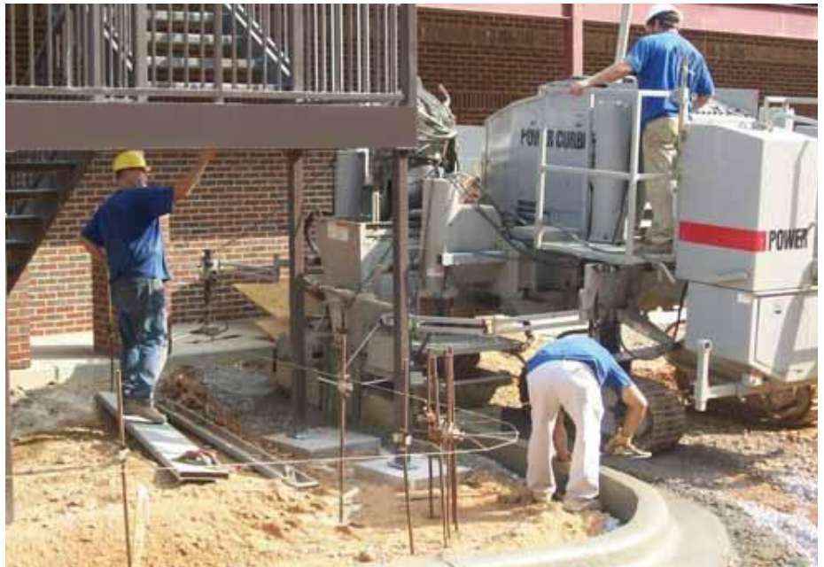
Machine maneuvers in tight areas, minimizing tie-ins.
