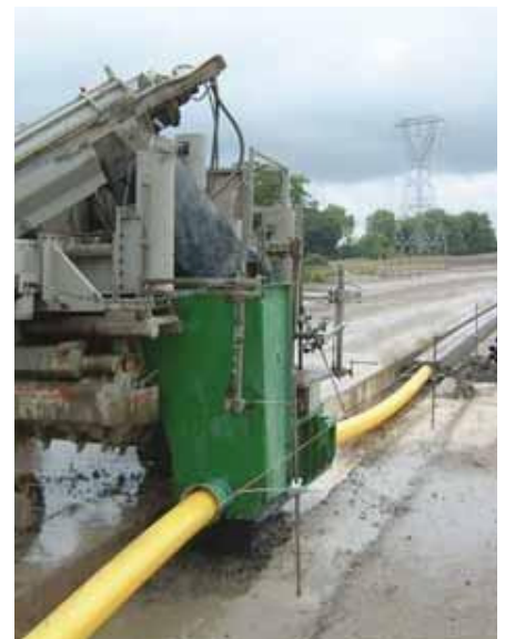
Slotted drain showing inflated tube.
