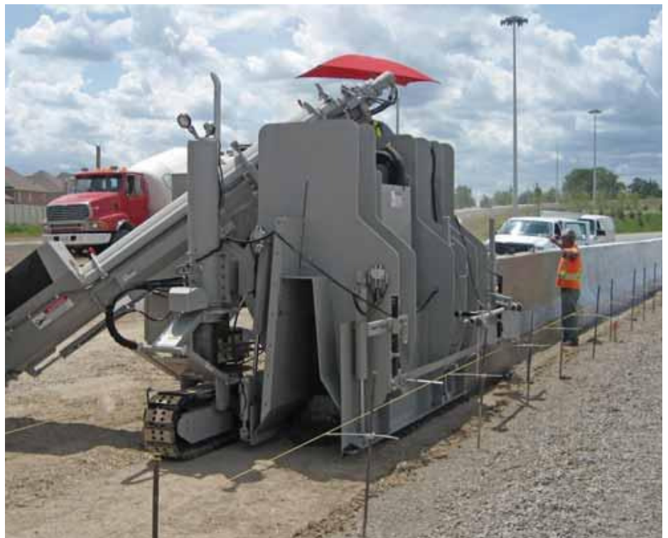
5700-C-MAX pouring large variable barrier wall.
