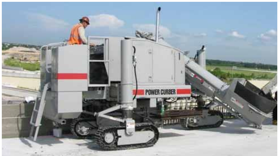
5700-C pouring bridge parapet in Florida.
