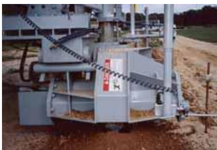
Custom trencher trimmer for footings.
