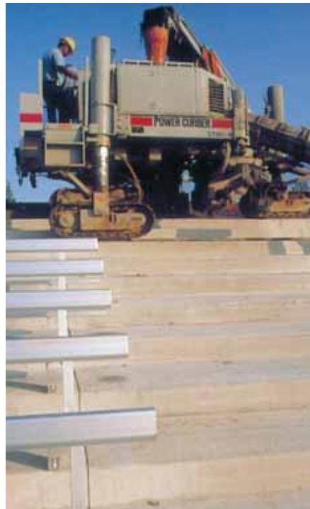
Machine runs on previous day's pour.
