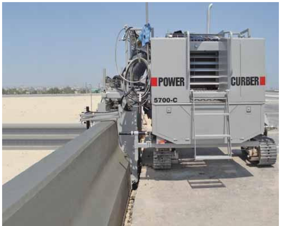
Barrier poured below grade, 49" (1.25m) tall.
