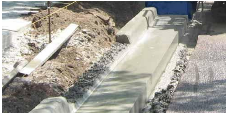
Driveway knives reduce wasted material and labor. Some hand finishing is required.
