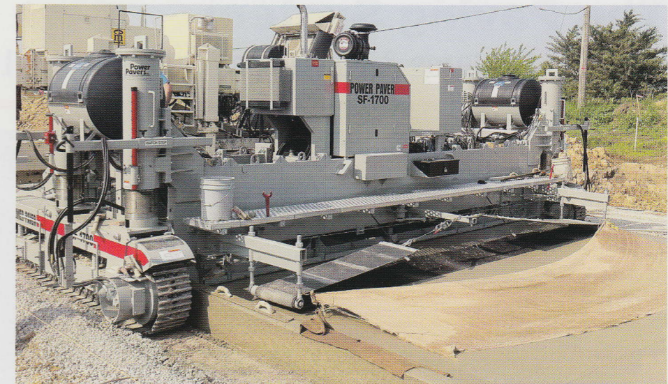
SF-1700 paving a street with optional integral curb. An optional belt finisher and burlap drag provide the desired finish.
