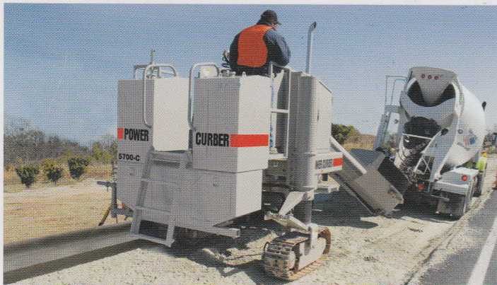
▲ Power Curbers 5700-C Slip-Form Curb Machine
