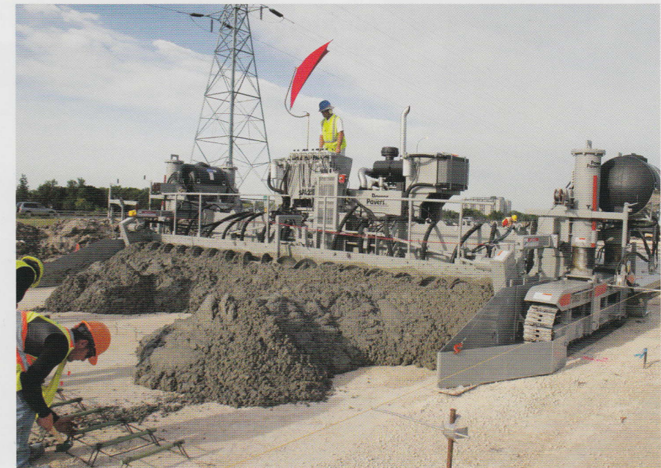
Front view of the SF-2700 paving over dowel baskets in Saskatchewan.
